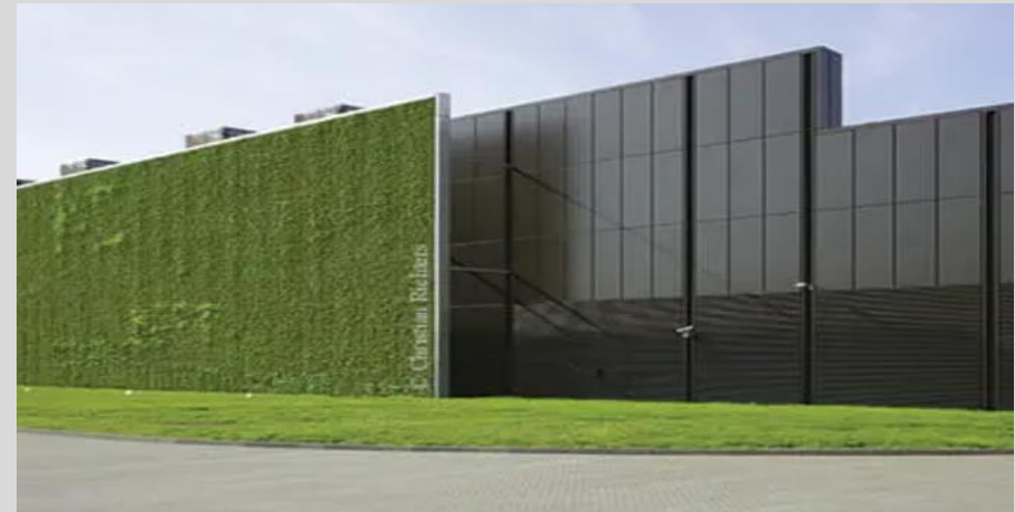
Citibank data centre, Frankfurt – Arup
